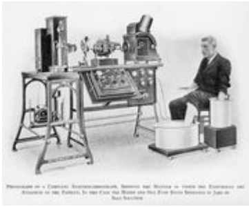
im6. ECG as done by Willem Einthoven Electromechanical technology [2]
