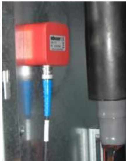
Figure 34: Method that were used for the TEV sensor installation
