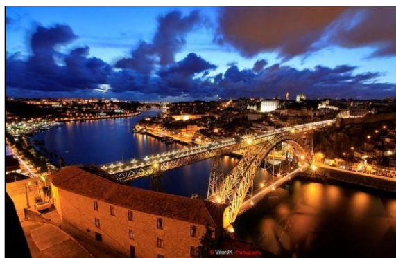
(β) Dom Luís Bridge, Porto, Portugal
