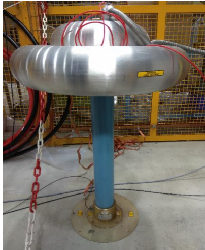
Εικόνα 43: The HV divider, with the toroidal conductor placed on top
