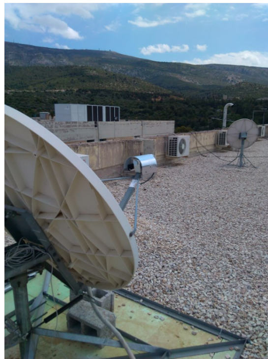
Figure 4-40: Back view of the antenna with the acrylic sheet installed around the LNB and feeder
