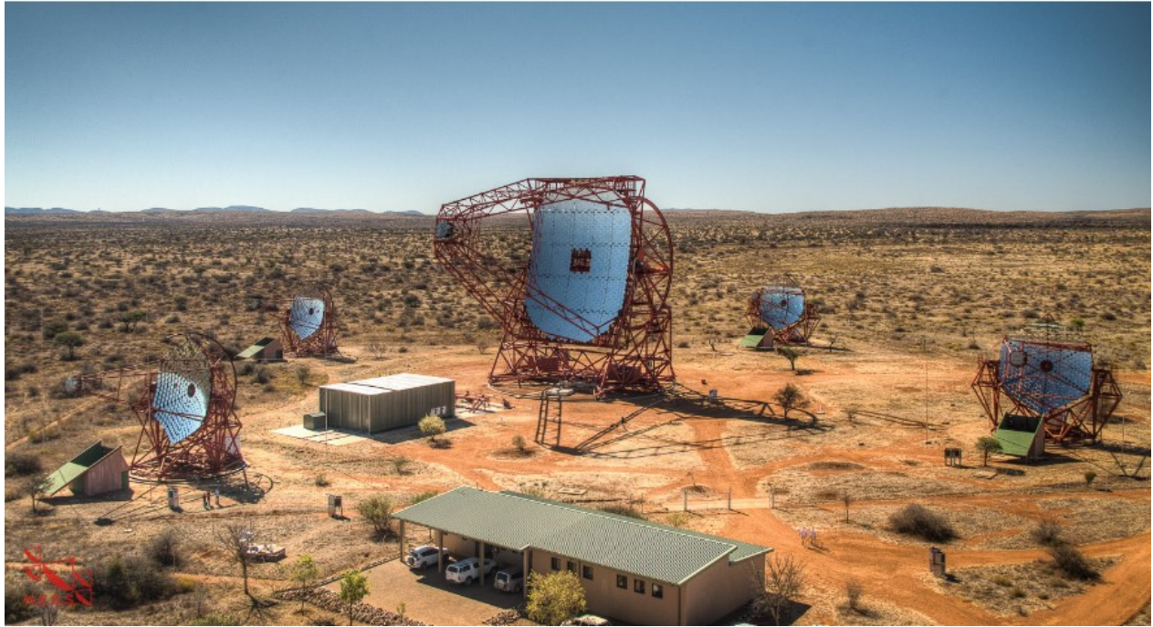
Figure 2.4.2: An overview of the H.E.S.S. array, with CT1-4 arranged in a square and CT5 in the middle. From [36].
