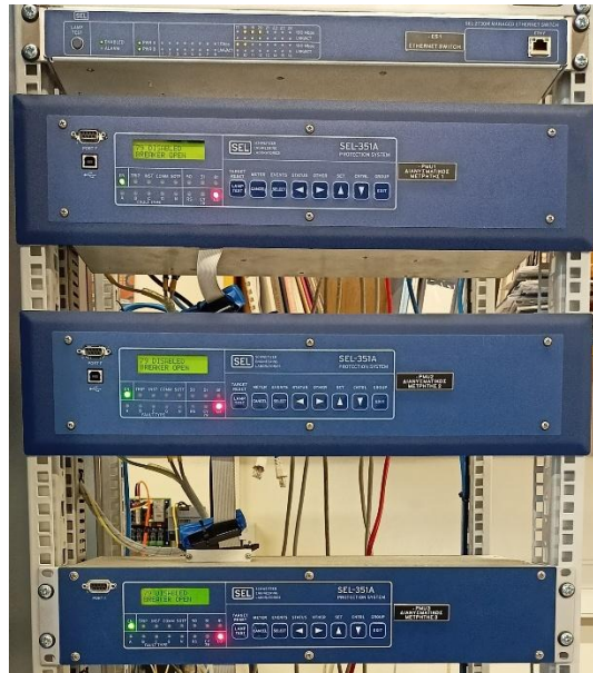
Figure 9.3: SEL-2730M switch and three SEL-351A PMUs.
